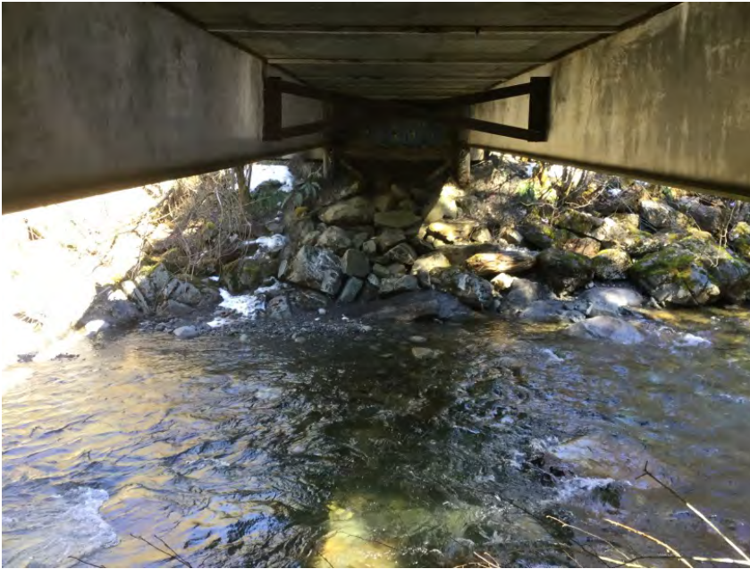
Right Bank Abutment when facing downstream
