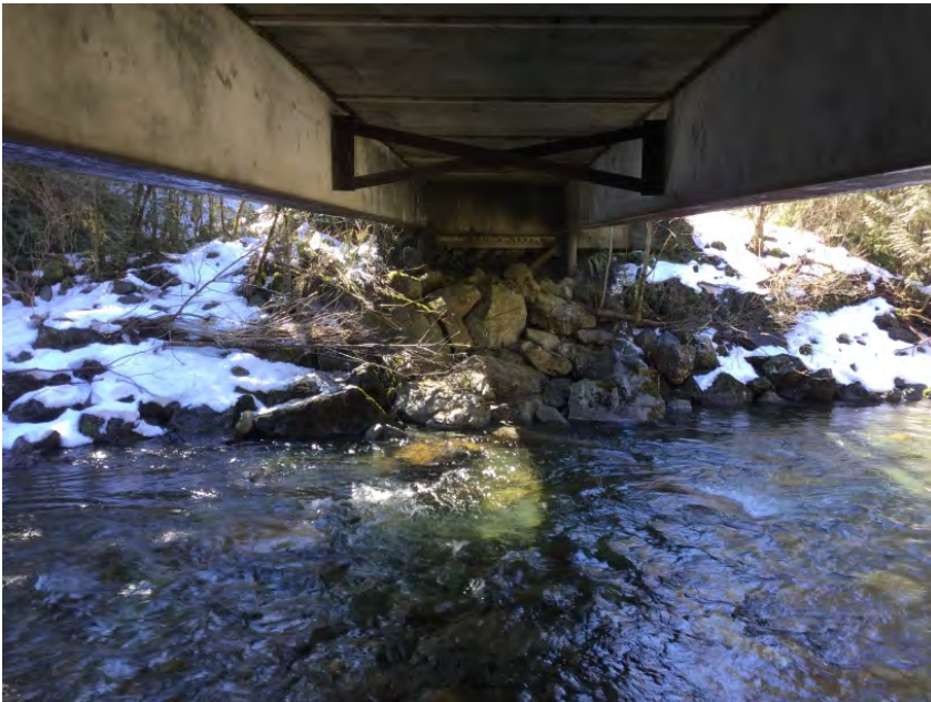
Left Bank Abutment when facing downstream
